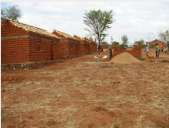
Built from locally manufactured clay brick, these Leper Houses are both functional and durable.
